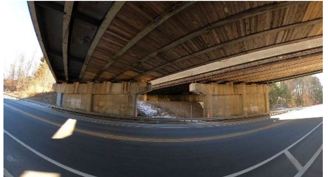
I-90 Mainline over MA-67 (Boston Road)
