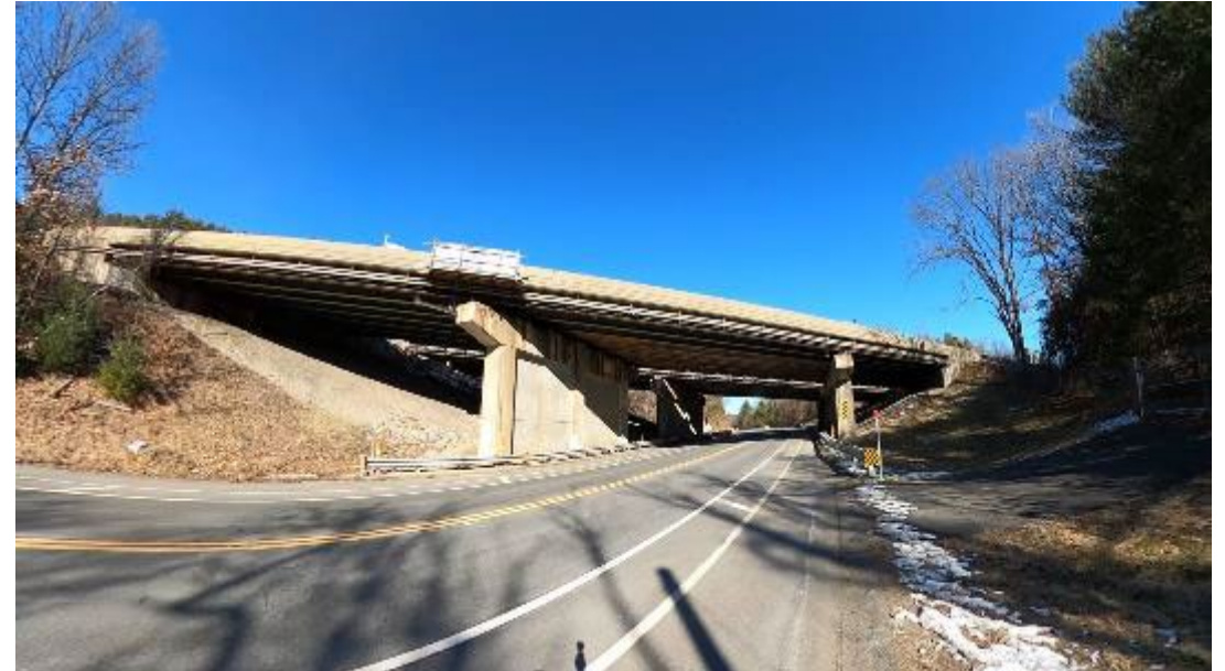
I-90 Mainline over MA-67 (Boston Road)
