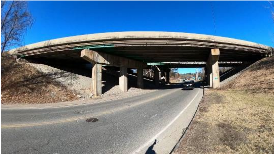
I-90 Mainline over MA-32 (Thorndike Street)
