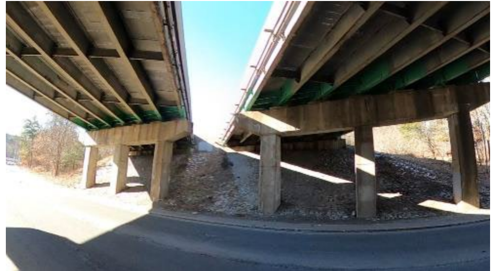
I-90 Mainline over MA-32 (Thorndike Street)
