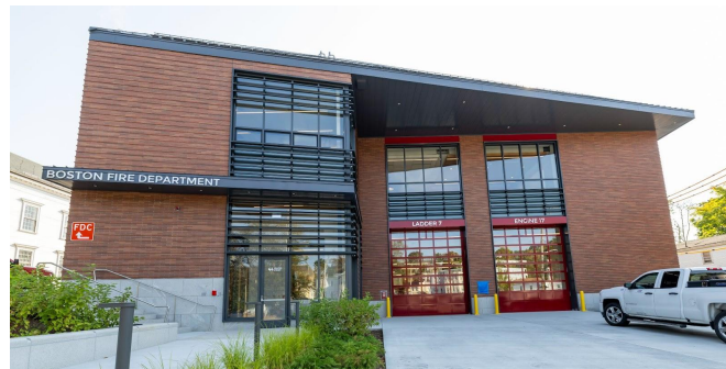
Engine 17 Fire Station
