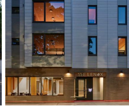
11 E. Lenox Street Boston MA Haycon Construction
