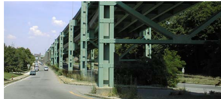
Fall River Viaduct
