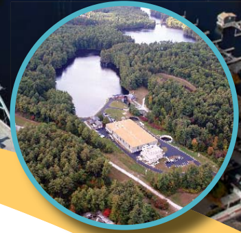
Fay, Spofford & Thorndike Pennichuck Water Works Integrated Water Treatment Plant Improvements
