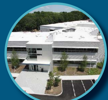
Weston & Sampson Engineers, Inc./ HKT Architects, Inc. New Public Services Facility Lexington, MA
