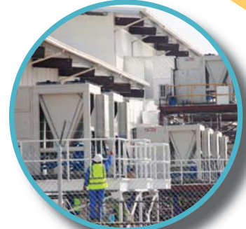
Tetra Tech US Forces – Iraq Operations Facility
